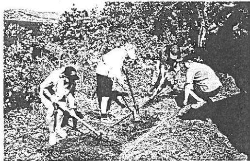
Clearing the old tramway track
